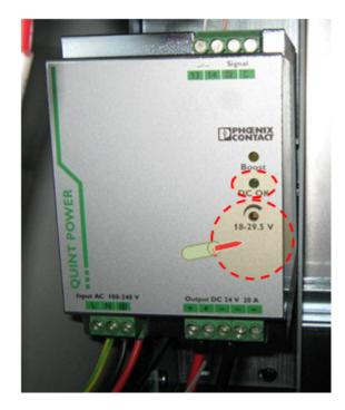
3 Connect the multimeter to measure DC output voltage of power supply 2 at the terminal block . See the following figure.
