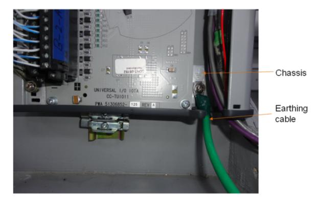
Figure 164: Grounding connections
